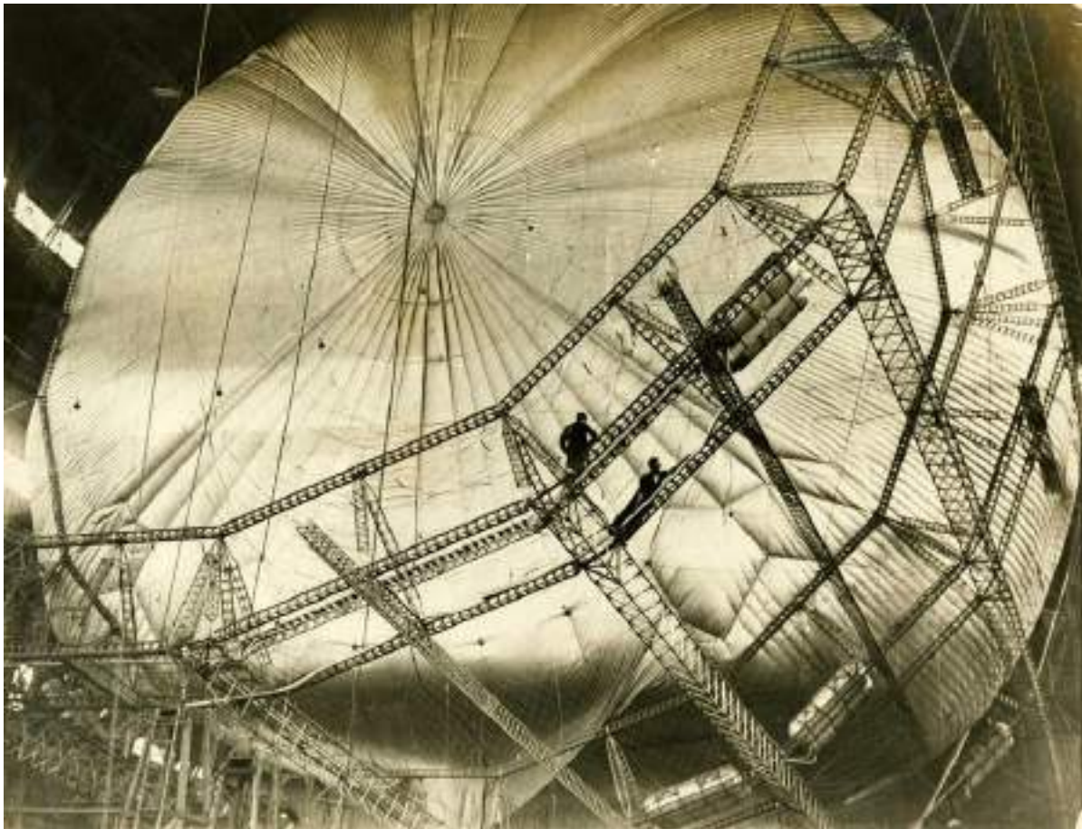
Figure 5 Gas bag within R.101 structure (the photograph shows a test bay mounted on the door of the airship shed at Cardington).
